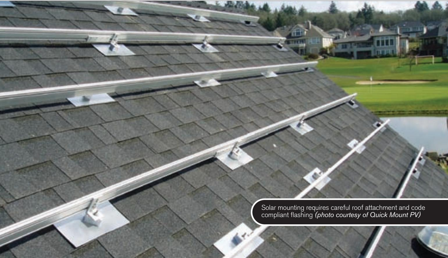
Solar mounting requires careful roof attachment and code compliant flashing (*photo courtesy of Quick Mount PV*)
